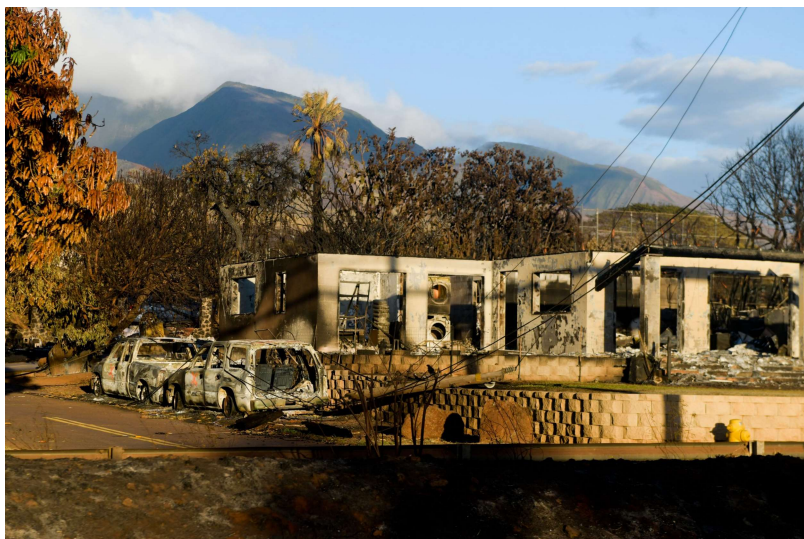
A wildfire destroyed the town of Lahaina, Hawaii, in August. PHOTO: ELYSE BUTLER FOR THE WALL STREET JOURNAL
